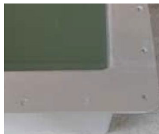
Ensure flanges are clean and free from grease, grit etc.
