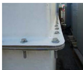
Some sealant may squeeze out from between the flanges. This is normal.
