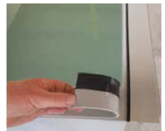
When applying sealant to the next flange ensure an overlap
