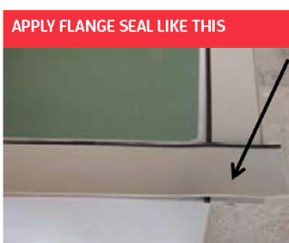
Flange sealant overlaps like this
